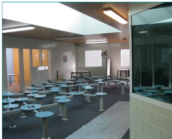
Figure 5: Visits room – being repainted
