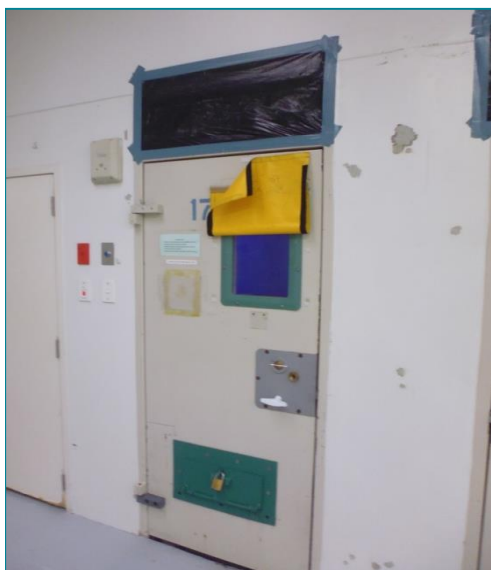
Figure 3: ARU—dry room entrance
