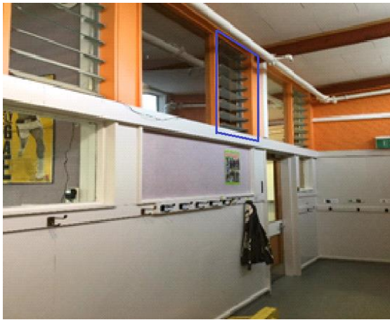
From corridor, June 2017 (photo: Ruru)
