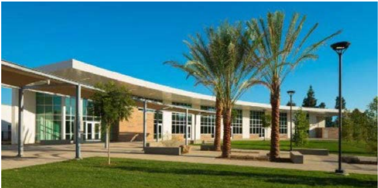
Las Colinas Detention and Re-entry Facility training and rehabilitation Unit
